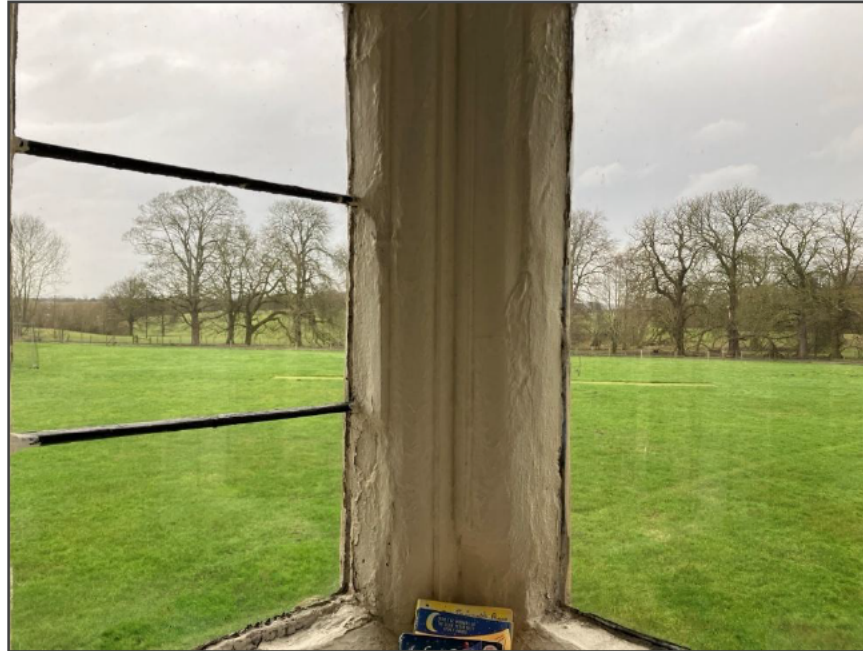
Plate 3: View from the lower storeys of the north elevation, looking north and north-west.
